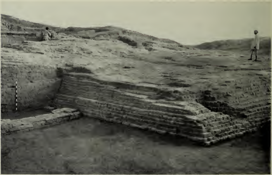
B. Kalibangan, Rajasthan: one of the mud-brick towers of the Harappan citadel (p. 22).
