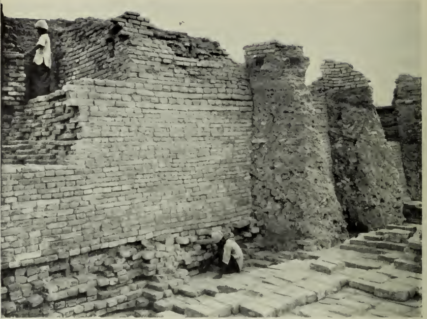
A. Mohenjo-daro: upper part of podium of Great Granary as seen from the loading-platform, showing late walls (on earthen supports) built when the ground-level had risen to the top of the podium (excavated 1950) (p. 127).
